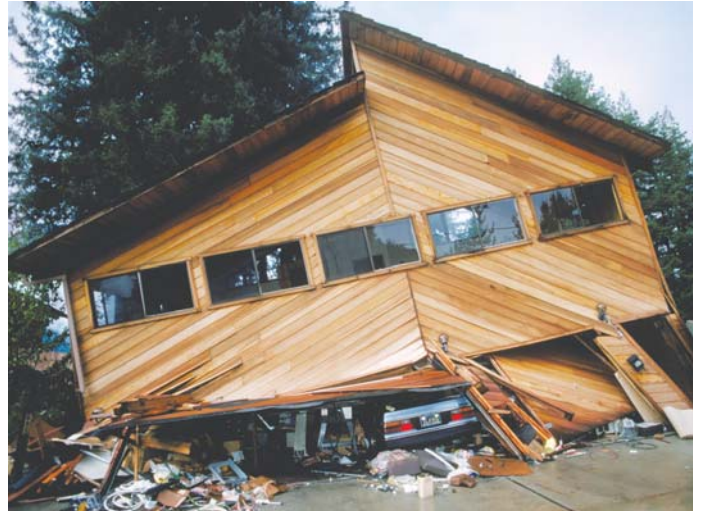
This home in the Santa Cruz Mountains collapsed in the 1989 magnitude 6.9 Loma Prieta earthquake (USGS photo).
