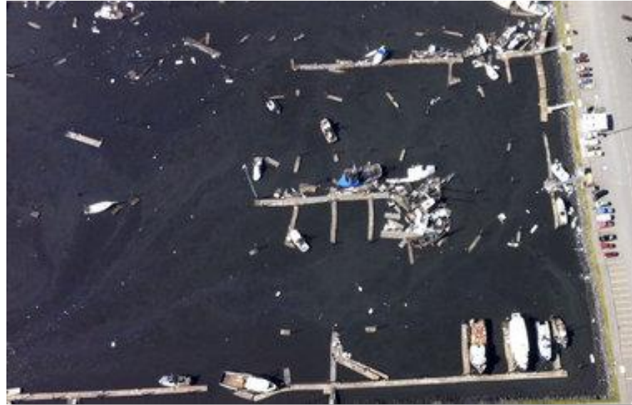
Crescent City Port, CA. Japan Tsunami on March, 2011.
